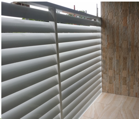
Frame can go all the way around the parameter and if the blade span is over 3000 a support in the centre is needed
