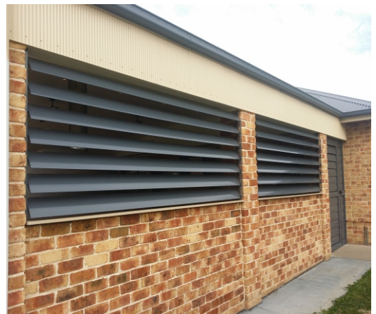
Mounted in a hole in the wall with side frame only
