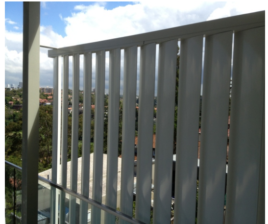
Frame less The 100x50 box frame can go on either end leaving sides open with blade only
